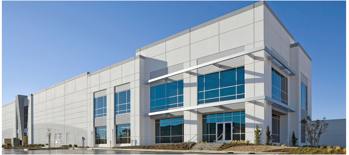
Unique COPE-Nano Building dedicated for the R&I activities in FPEs & Nanotechnologies, its state-of-the-art research infrastructure (clean rooms, advanced equipment, facilities and pilot lines), and its legal, administrative and management activities
